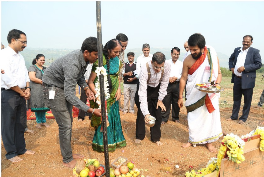
Ground-breaking of IIMB's second campus in Jigani hobli of Anekal taluka with Prof. R. Srinivasan (Director in Charge), 21st October 2016.
